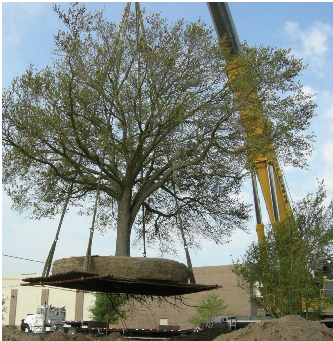
Relocating 24-inch caliper live oak at Keesler Air Force Base (AFB) in Mississippi
