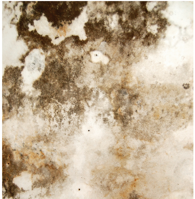
Mold inside of ceiling tile
